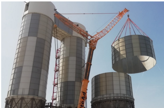
This setup only requires four horizontal connections per silo, for a perfect sealing of each unit.
