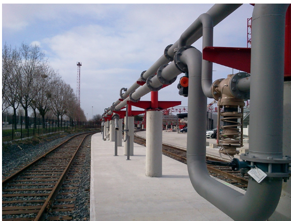
The train unloading area is served by multiple inlets that reduce down to one manoeuvre required for positioning.
