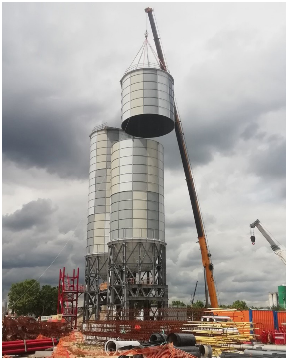
Having long vertical panels with limited horizontal flanges reduces the need for operations at height and the overall number of bolts.
